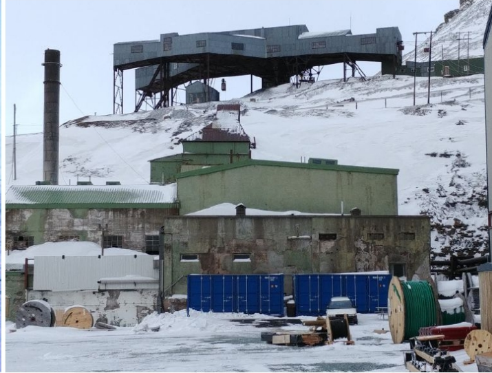
The old central transport hub for coal and coal-fired power station. Photo: Dina Brode-Roger.
