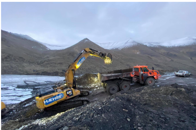
Figure 5: Dismantling of Svea 1. Photo: Ranghild Utne Bekkeheien.
