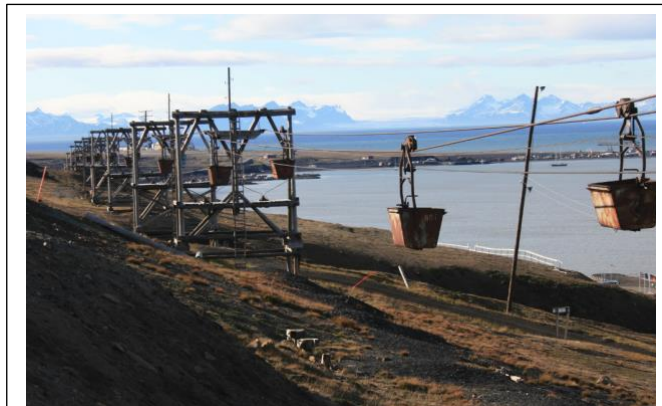
Figure 7.11 The cable car system for transporting coal is a dominant cultural heritage feature in Longyearbyen (Photo: NIKU)
